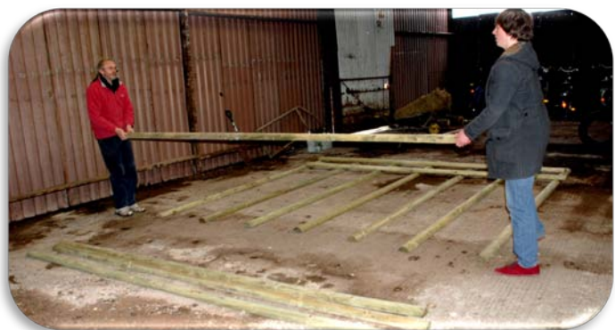
Willow Bridge Eco Gym - laying a workout grid
